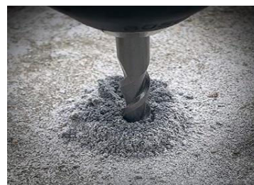
Figure 43: Time taken to drill hole into asphalt was measured
