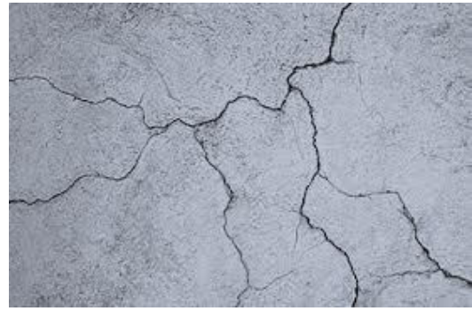
Figure 45: Hammering the 20g asphalt mixture resulted in cracking
