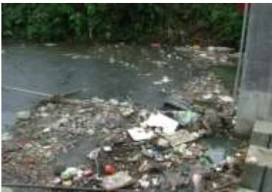
(取水閘門前漂浮的垃圾)
