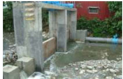
(取水閘門及管道)
